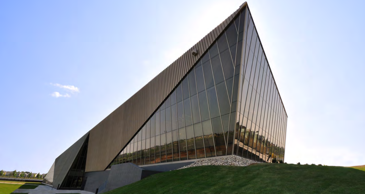
Clareview Community Recreation Centre and Library | Edmonton, AB CISC Alberta Steel Design Award Finalist - Building Communities | 2015
