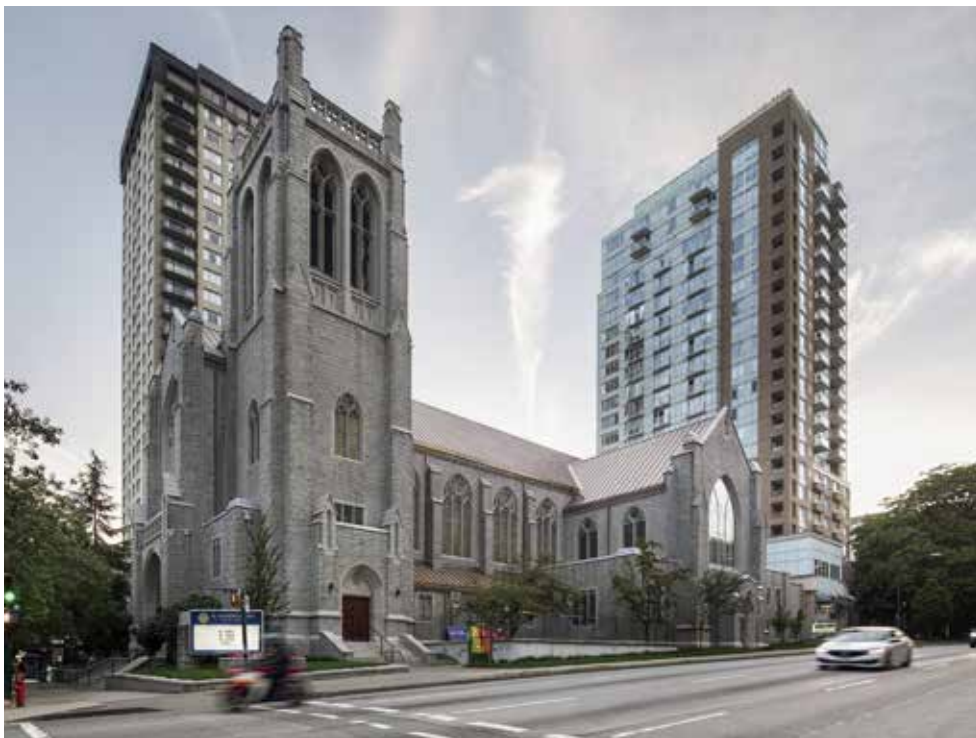
Top: St. Andrew's-Wesley United Church (restoration and upgrade) Bottom: Parkade restoration work
