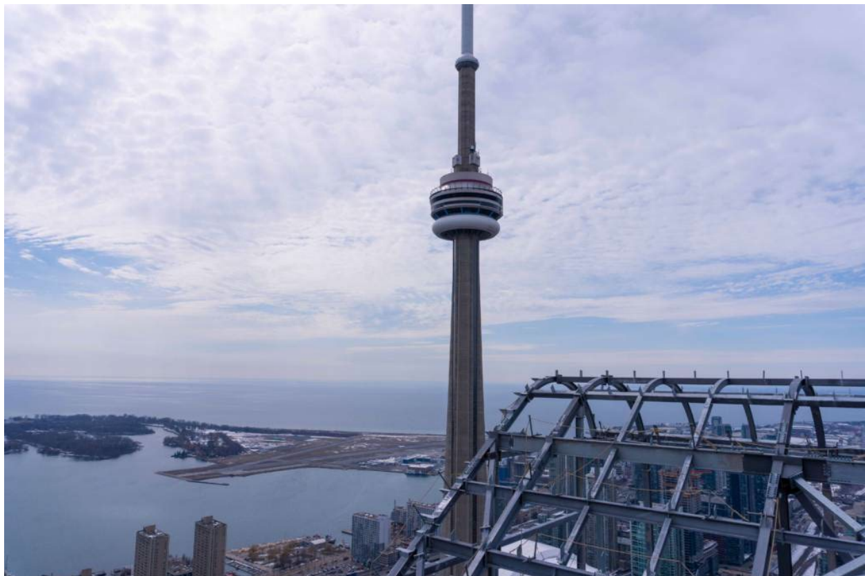
Image 2 of 4 - A view of the structure with CN Tower in the background.
