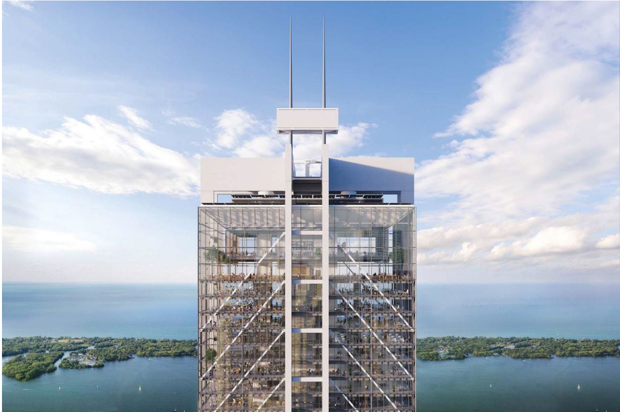
View of the upper floors and crown of the HUB, image from submission to City of Toronto
