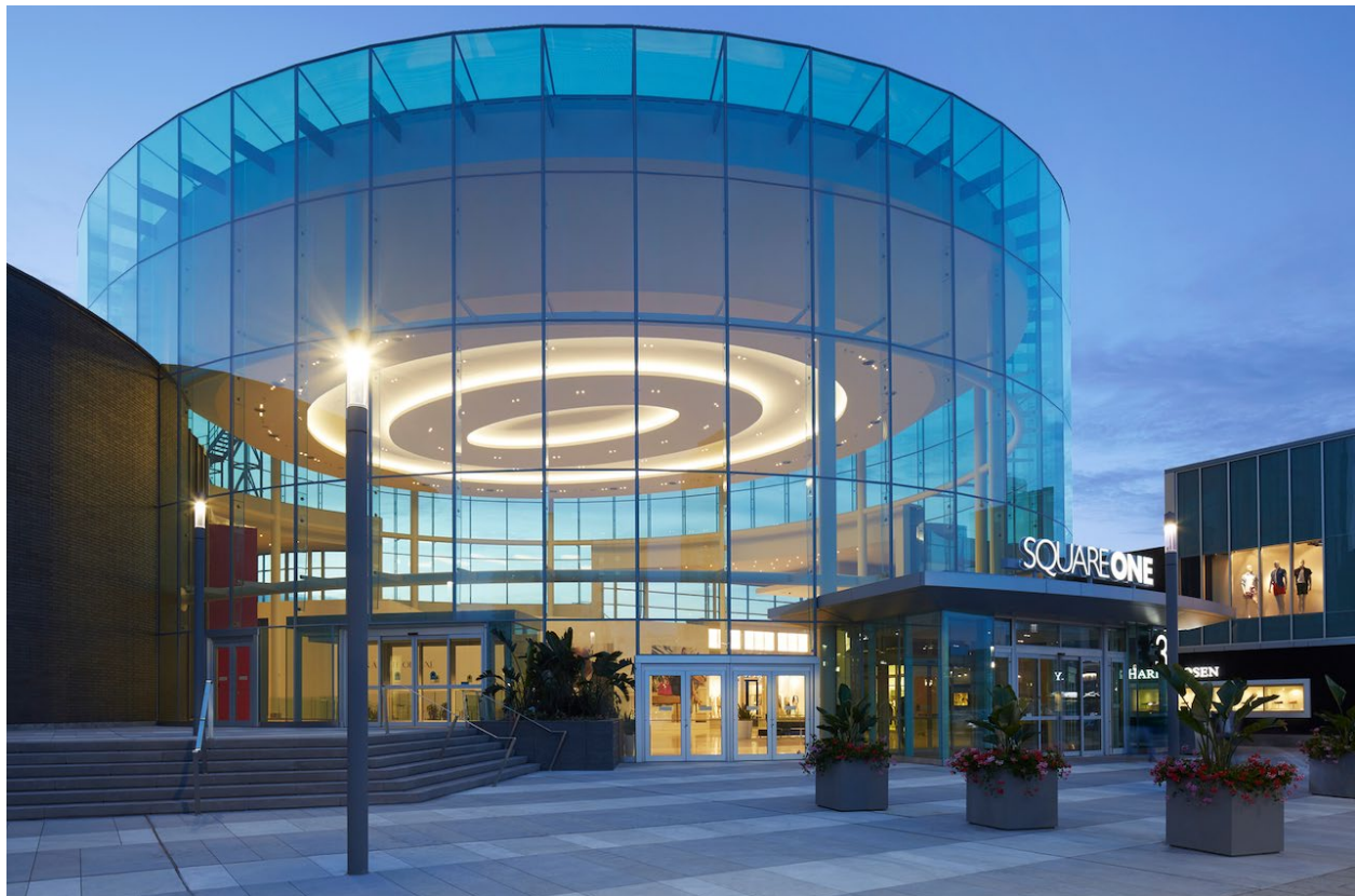
The Rotunda entrance at Square One Shopping Centre, image courtesy of RJC Engineers
