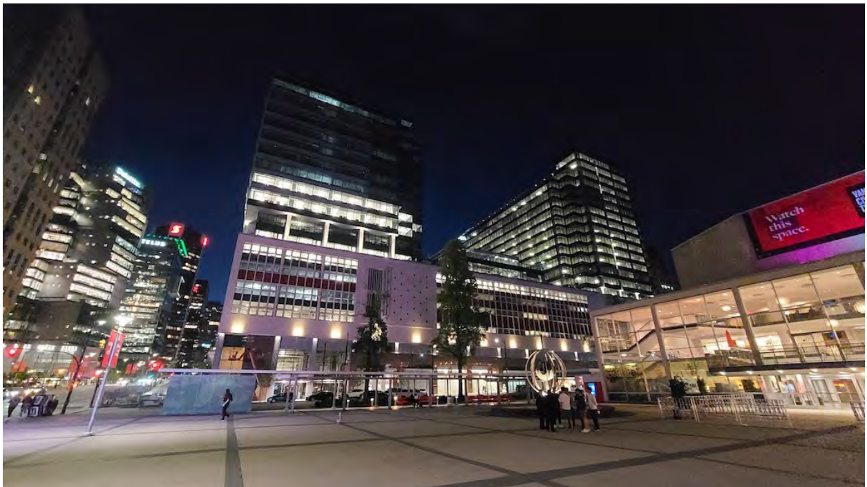
Exterior of The Post; Construction progress as of May 23, 2023. (Kenneth Chan/Daily Hive)
