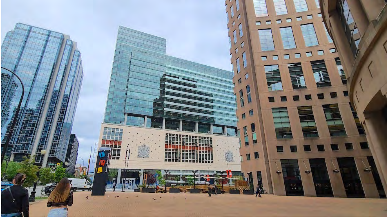
Exterior of The Post; Construction progress as of May 23, 2023. (Kenneth Chan/Daily Hive)
