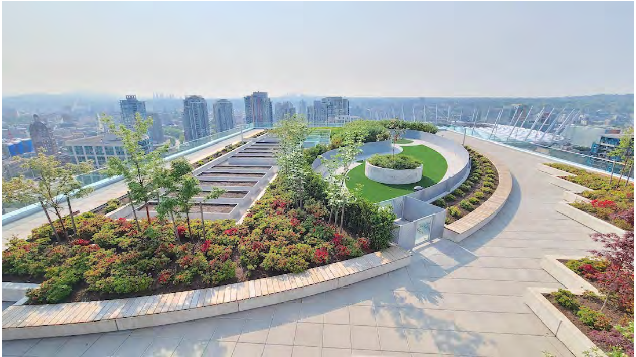
South Tower rooftop of The Post; Construction progress as of May 23, 2023. (Kenneth Chan/Daily Hive)
