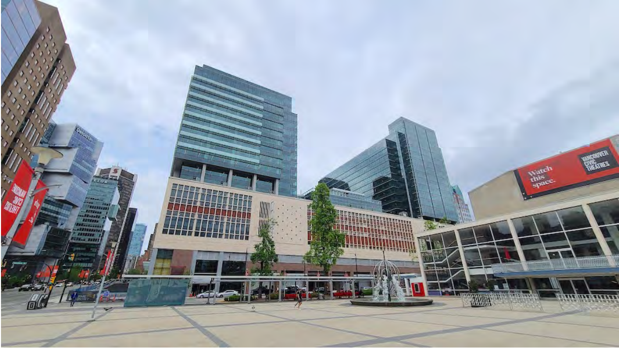
Exterior of The Post; Construction progress as of May 23, 2023. (Kenneth Chan/Daily Hive)
