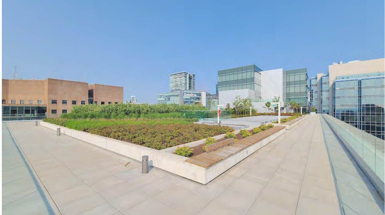
South Tower rooftop of The Post; Construction progress as of May 23, 2023. (Kenneth Chan/Daily Hive)
