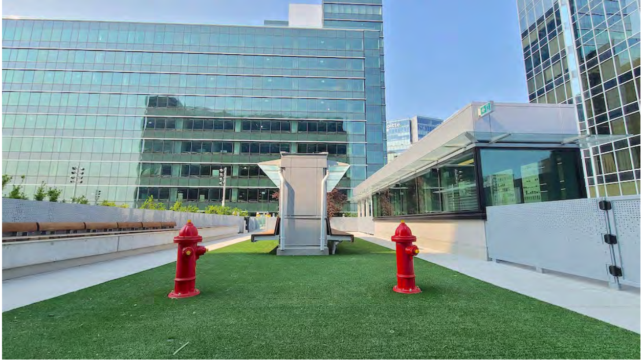
Dog park on the lower rooftop of The Post, between the North and South towers; Construction progress as of May 23, 2023. (Kenneth Chan/Daily Hive)
