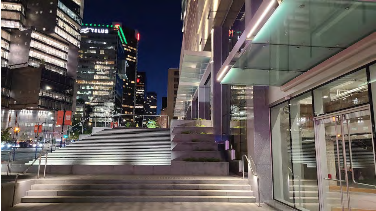
West Georgia Street public plaza; Construction progress as of May 23, 2023. (Kenneth Chan/Daily Hive)
