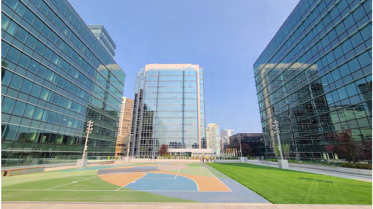
Full basketball court on the lower rooftop of The Post, between the North and South towers; Construction progress as of May 23, 2023. (Kenneth Chan/Daily Hive)
