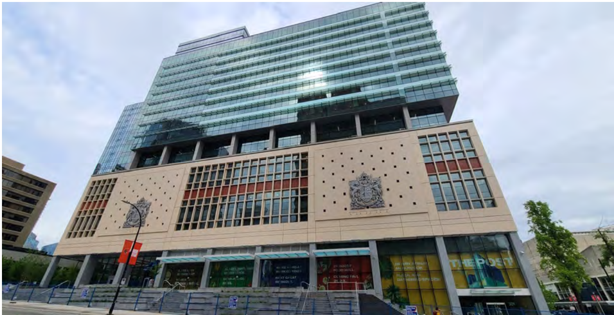
Exterior of The Post; Construction progress as of May 23, 2023. (Kenneth Chan/Daily Hive)
