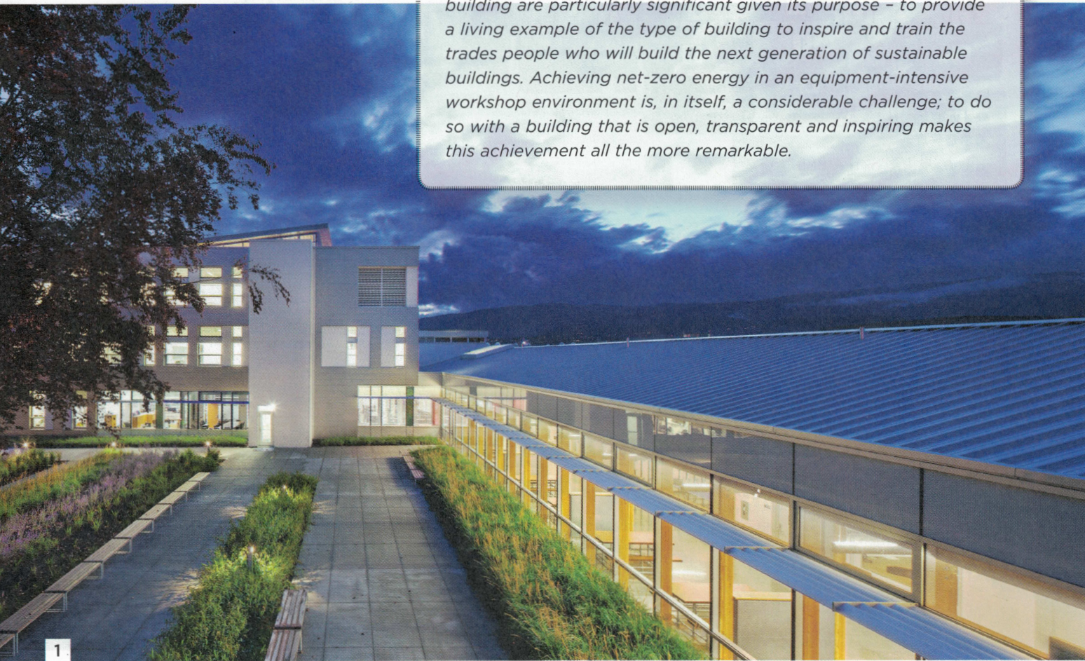
1. Looking east to the new addition and courtyard with view into corridor link. Exterior sunshades were provided by McGill Architectural Products .
